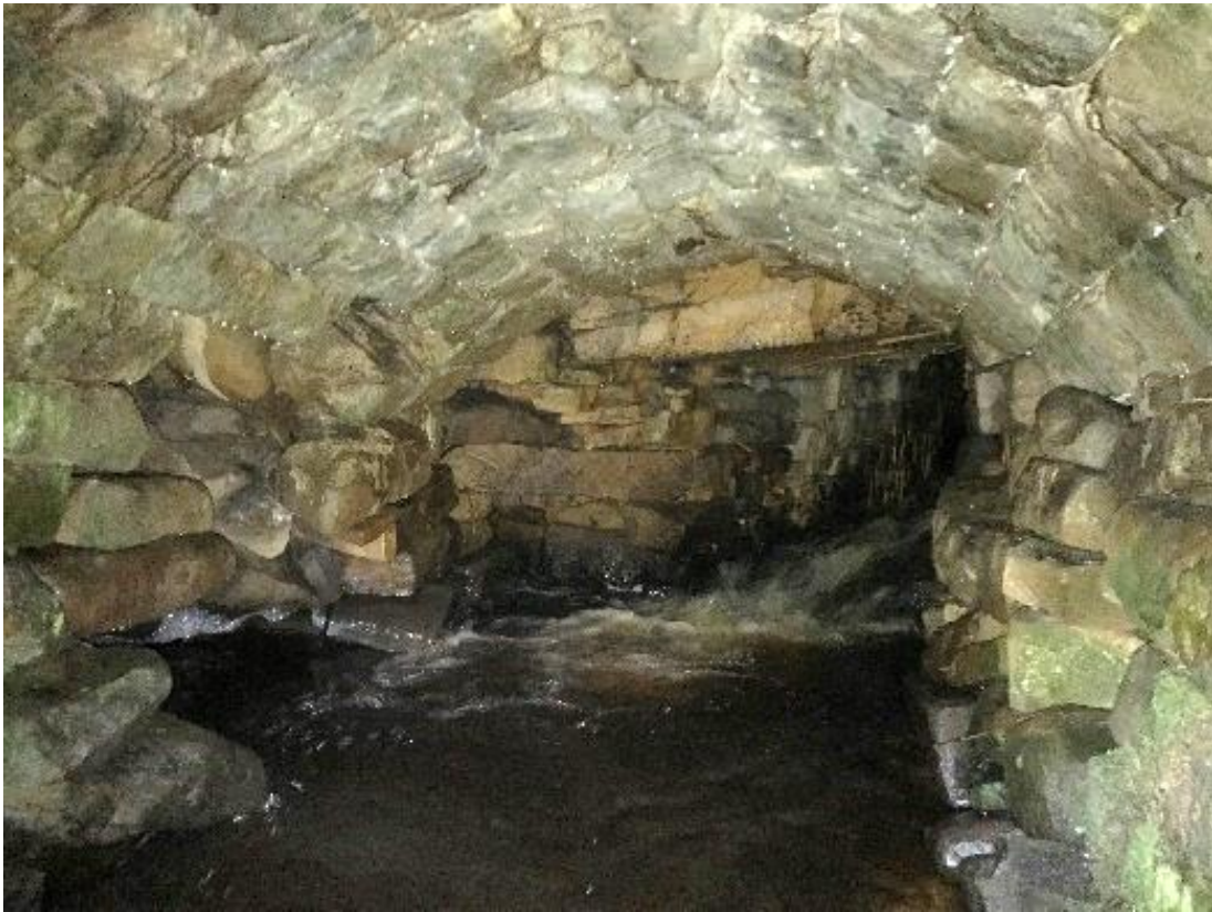
Photograph 8 – Photograph of the brick masonry arch at the culvert exit
