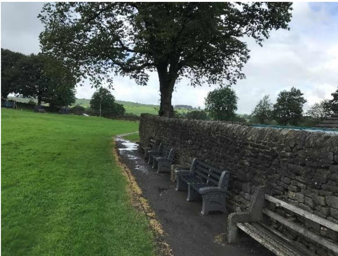
Photograph 6 – Standing water on the path leading to the tennis courts
